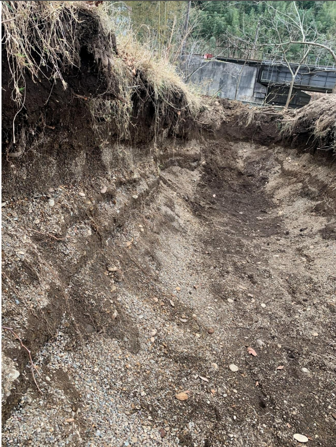
Fig. 12. Evaluation trench N1 after excavation
