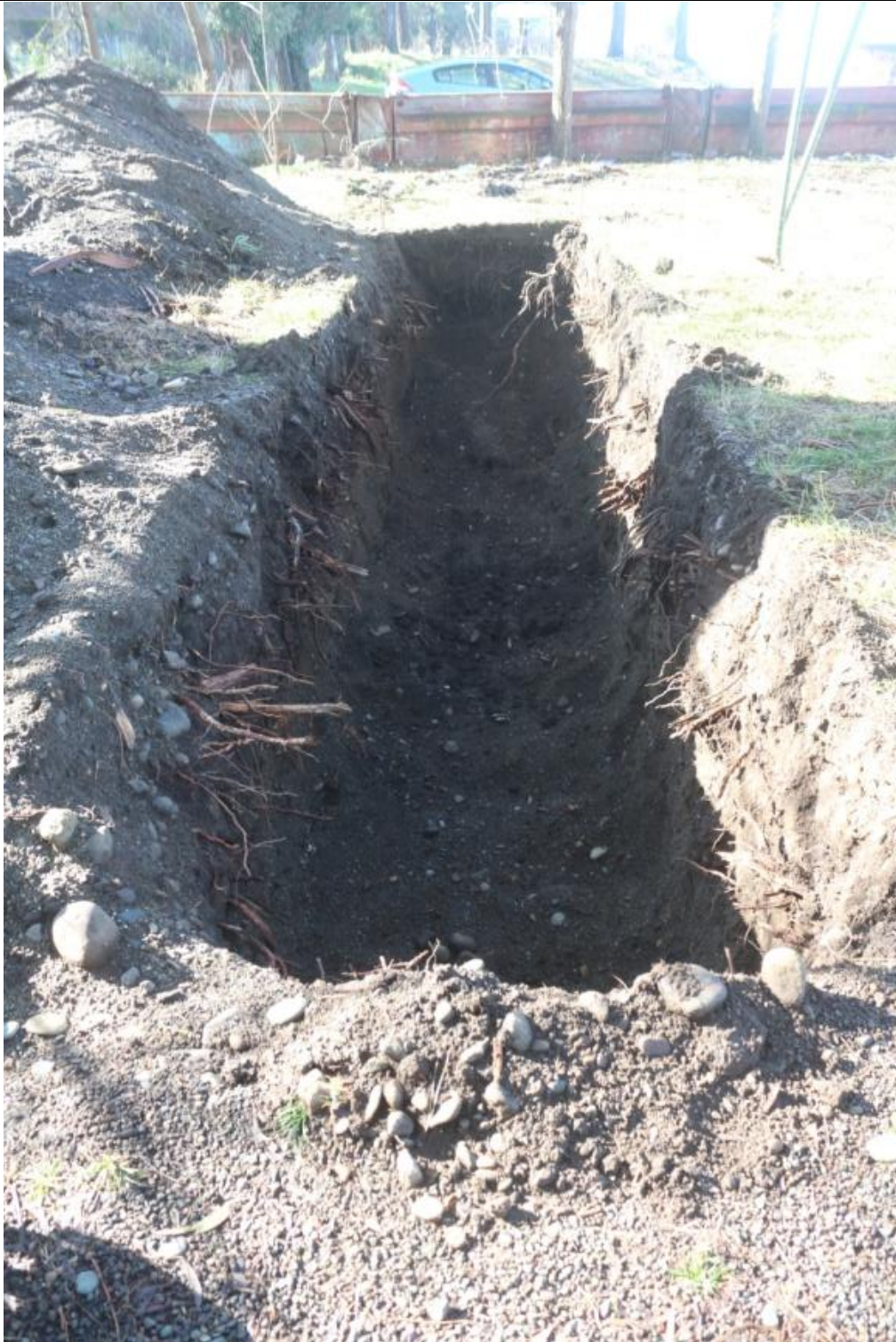
Fig. 13. Evaluation trench N2 after excavations
