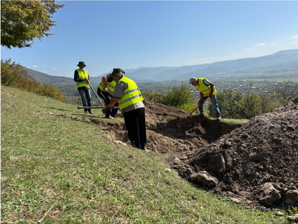
Trench N4. Working process
