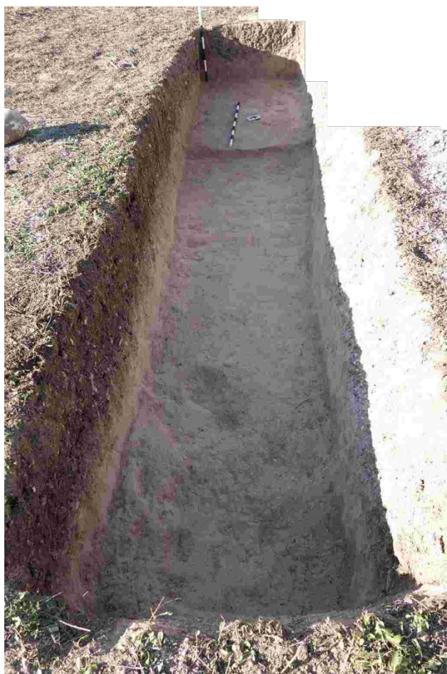
Pic. 11. T12 trench N7
