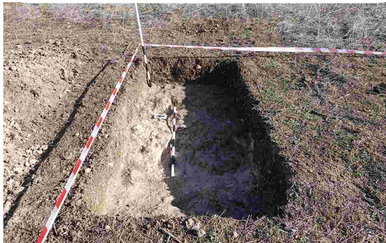
Pic. 5. T12 trench N1
